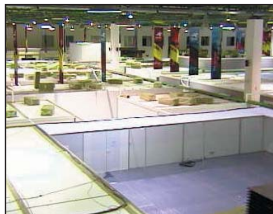
Construction and fit-out of the IBC has reached completion as DAGBS prepares for the arrival of the first Rights Holders
