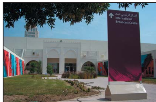
The east entrance of the International Broadcast Centre
